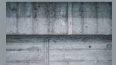
Original 1960s concrete ceiling with the formwork (wood grains) still visible. With the Downtown home style we have chosen not to hide this but to show off this special part of the building's history. This can also be finished if required.
